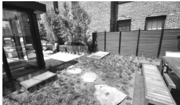
under construction - install by Plant Specialists
