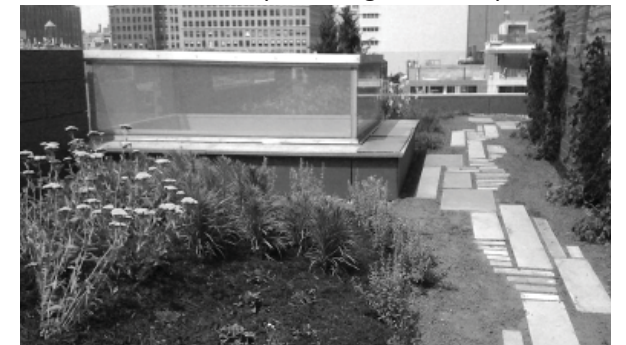
planting and paving install by Future Green Studio
