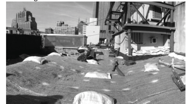
under construction - Hydrotech green roof system
